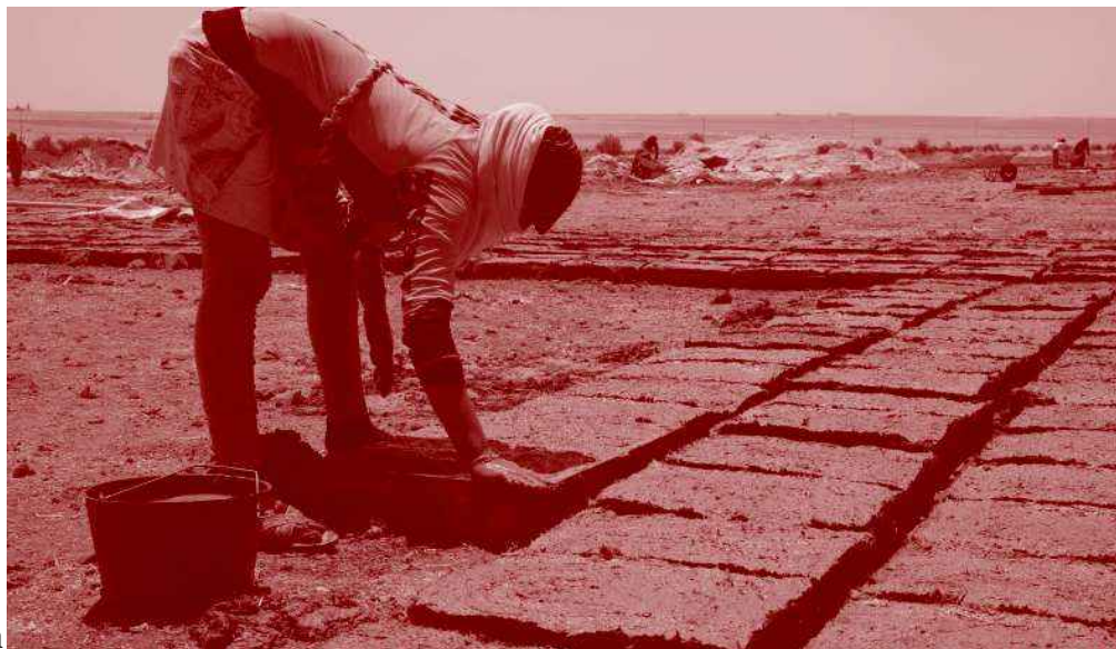
Construction starts on a women's center. Pic. Media Team, Jinwar.
